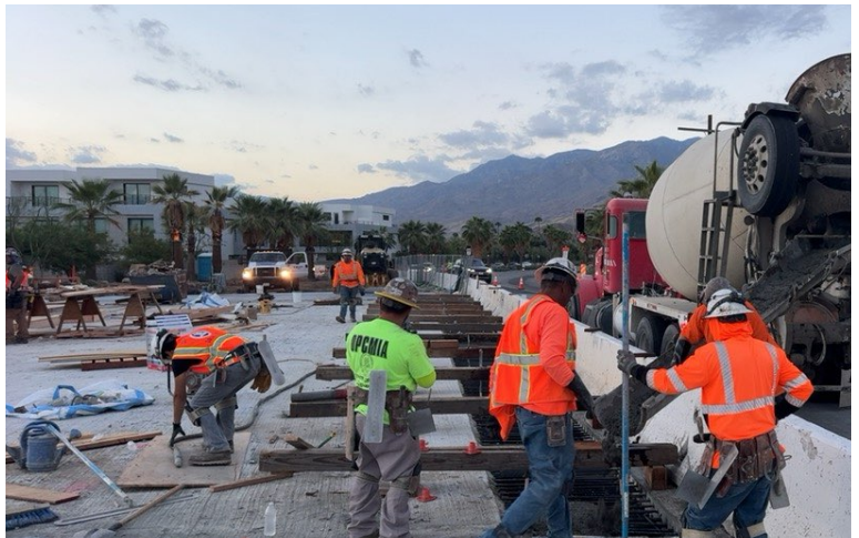
Crews are placing concrete for the center section of the bridge, connecting the new eastern and western spans to create one continuous bridge.
