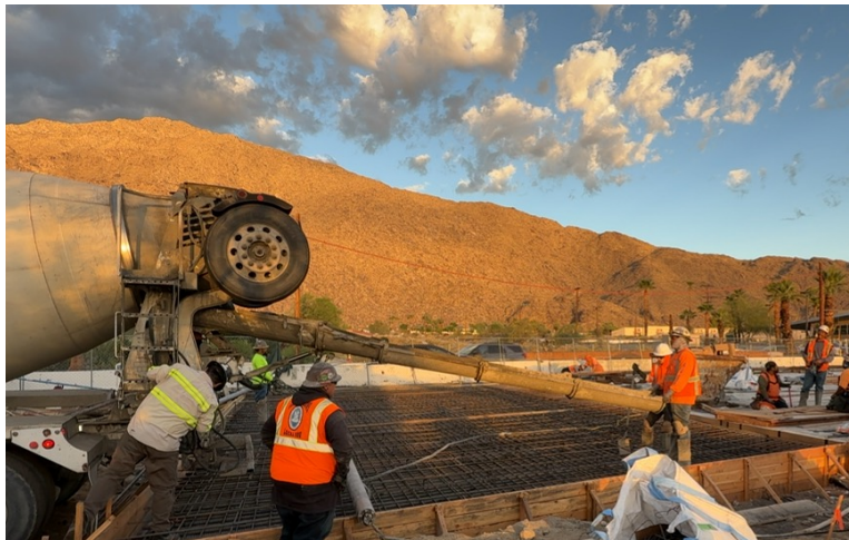
Crews are placing concrete for the eastern bridge approach, the section of roadway that connects the new bridge to South Palm Canyon Drive.
